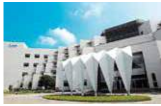
Tainan Plant (Diamond-rated Green Building)
